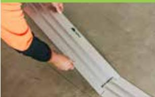
3. Chalk line the area you wish to cut. Lay the Sawtrac aluminium track/guide in line with the chalk line.
